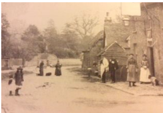
Church Street 1907 photo P Lipson
